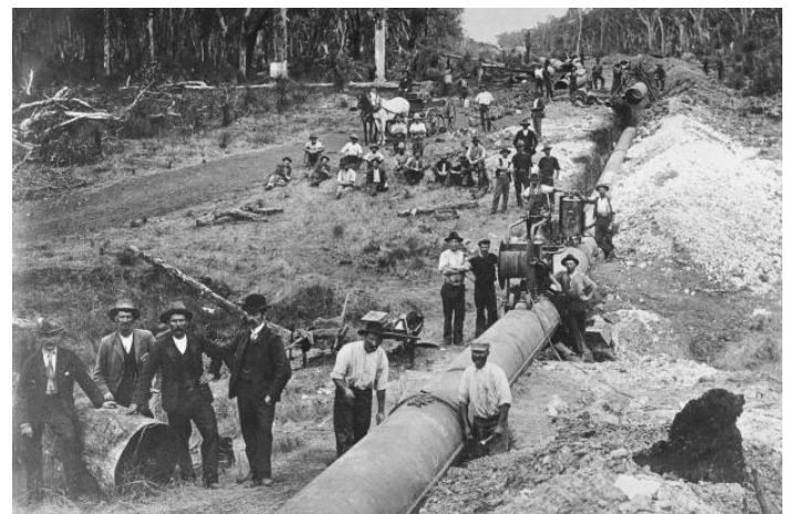
Construction of the Goldfields Pipeline
