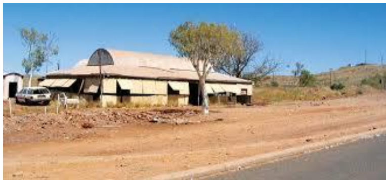
The ruins of Mt Welcome station, where the Withnell’s weathered the 1872 cyclone.
